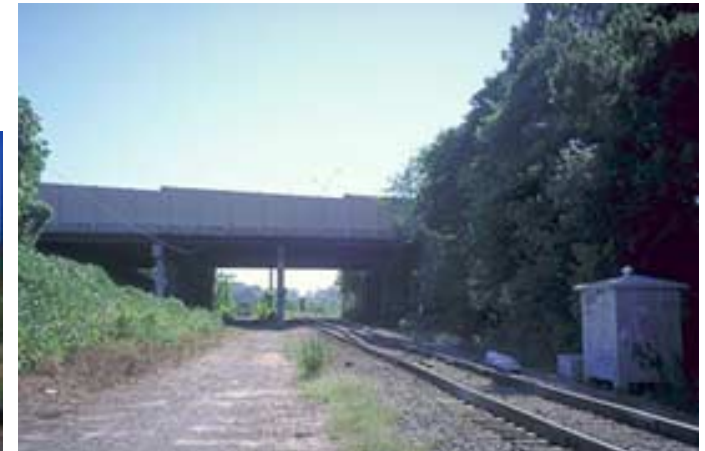
Crosses under I-75
