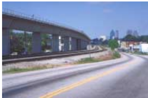
The belt line tunnels under this main line going into downtown
