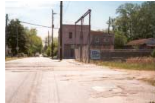
Crossing Wylie at grade
